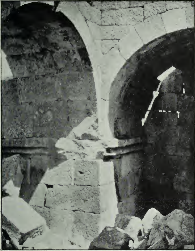
FIG. 202.—Mahaletch, interior angle of nave and N. transept.
